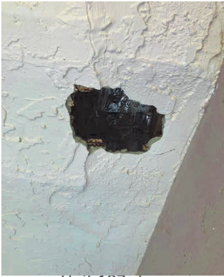
11 Unit 107 stucco removed to verify traming memebers
