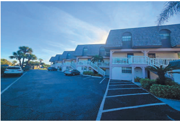
1 Front of Building 2 Units 105-109 & 209-218
