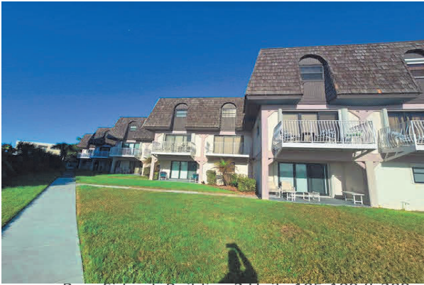
3 Rear Side of Building 2 Units 105-109 & 209-218
