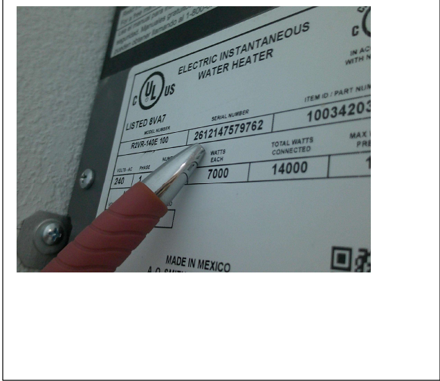
Water Heater Data Plate (2026)
