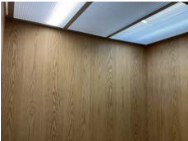
Cab wall finishes
