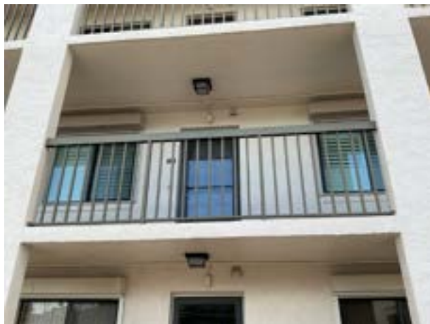
Railing finish fade
