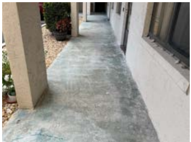
Concrete restoration ongoing
