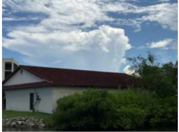
Metal roof at clubhouse
