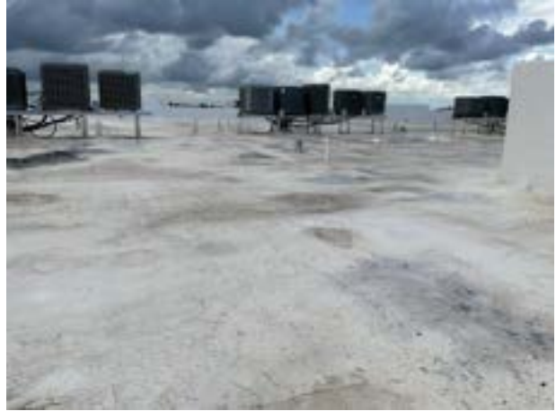
Foam roof overview
