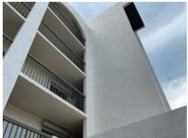
Stucco wall finishes
