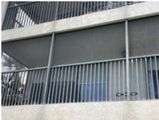
Aluminum railings with integrated screen frame
