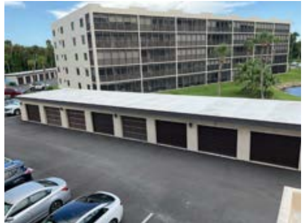
Foam roof overview
