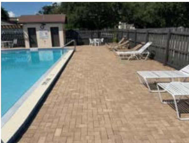
Paver pool deck overview
