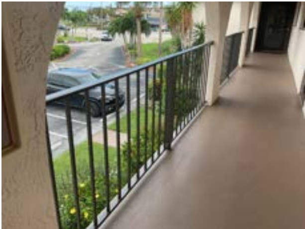
Railing finish fade
