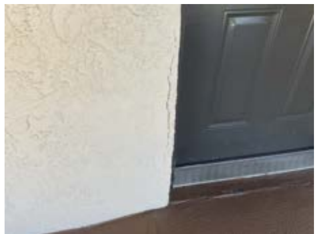
Stucco cracks
