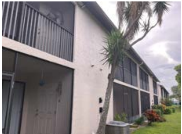
Stucco wall finishes
