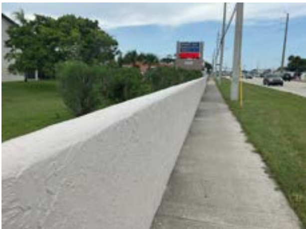
Perimeter wall paint finishes
