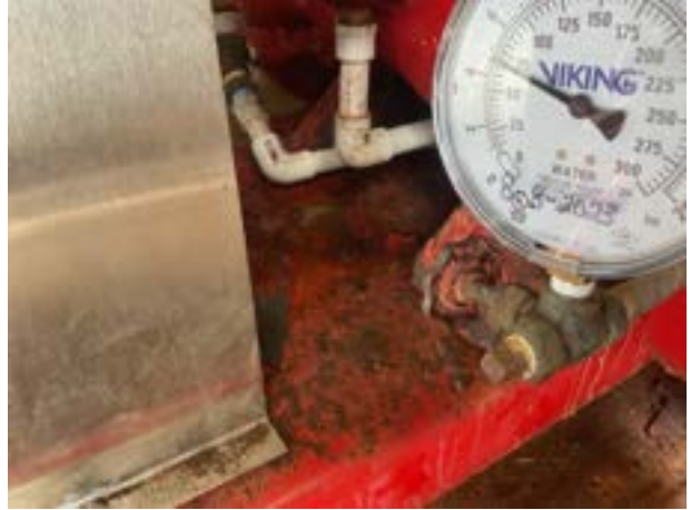
Water leaking
