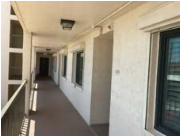
Stucco wall finishes at breezeways
