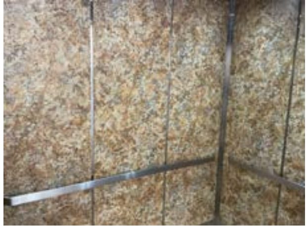
Renovated cab wall finishes
