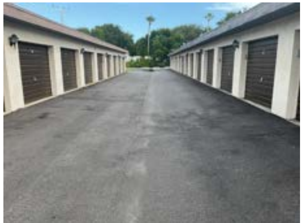
Pavement at garages
