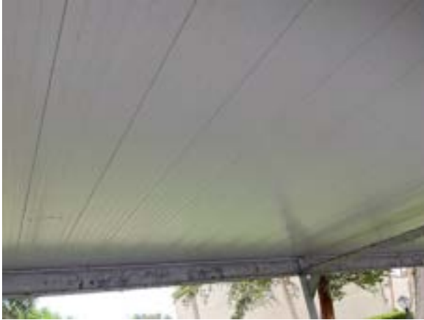
Carport under side
