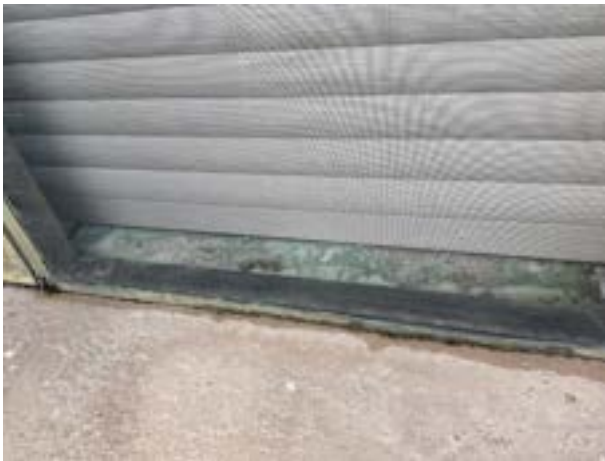
Coating deterioration
