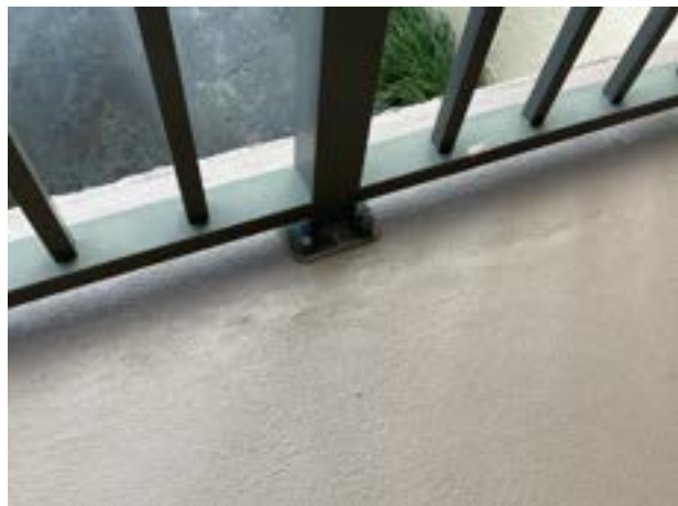
Mechanically attached railing post
