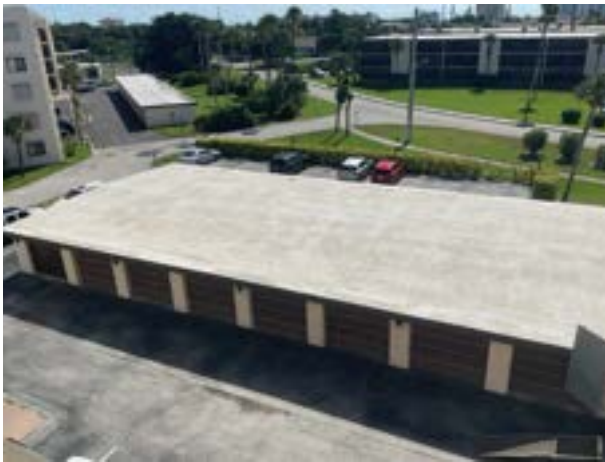
Foam roof overview
