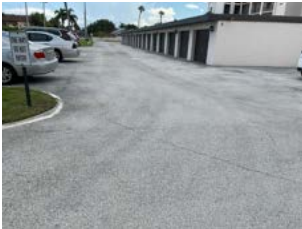
Pavement overview at building 9
