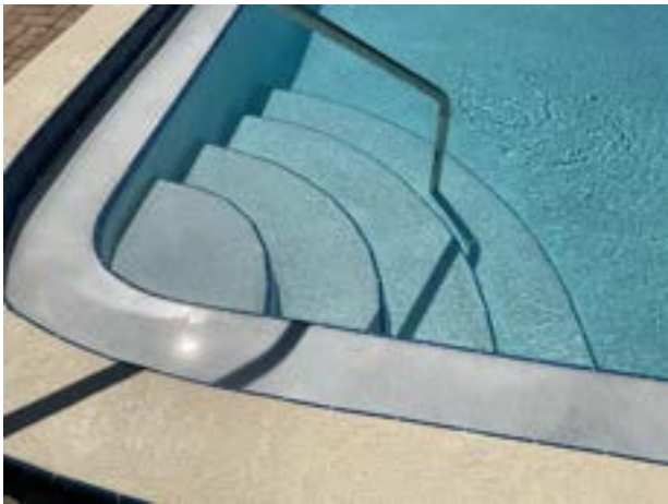
Plaster and tile finish at steps
