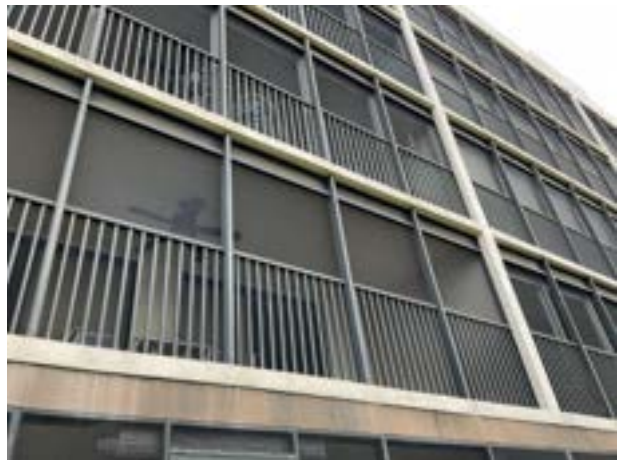
Aluminum railings with integrated screen frame
