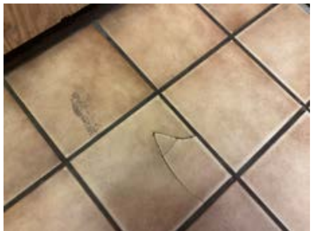
Tile cracks
