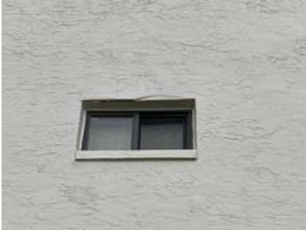
Stucco cracks
