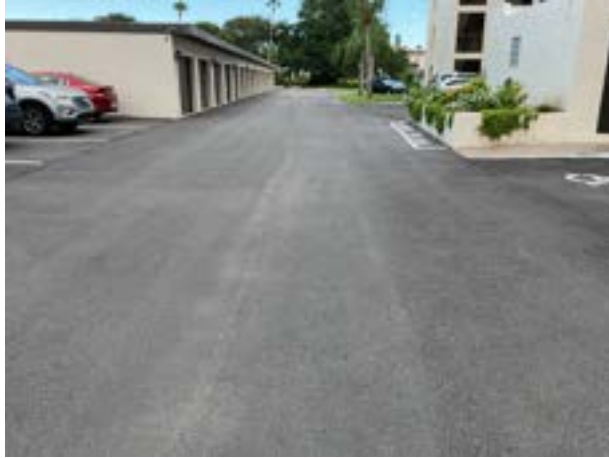
Pavement at 5 story buildings 10-12
