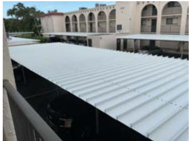
Carport metal roof
