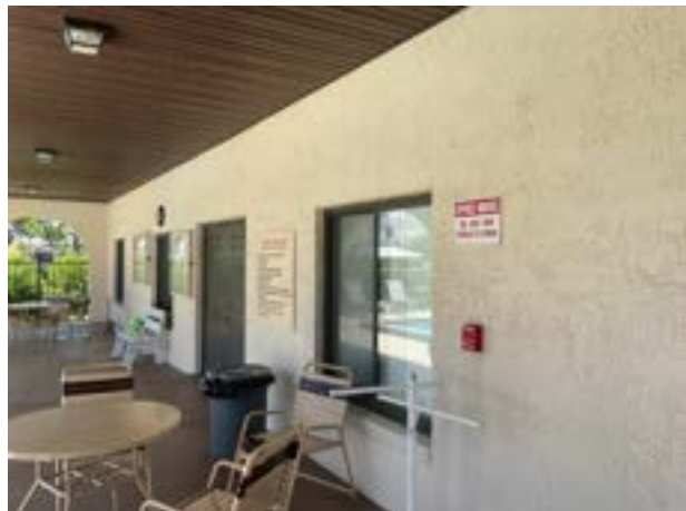
Windows and doors at clubhouse
