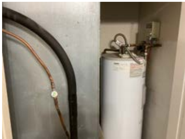
Air handling unit at clubhouse
