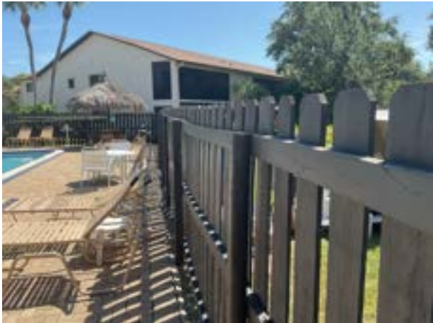
Wood fence overview
