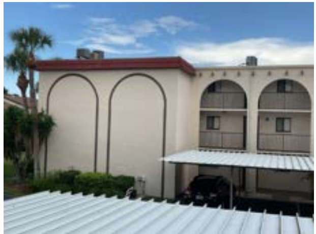
Stucco wall finishes
