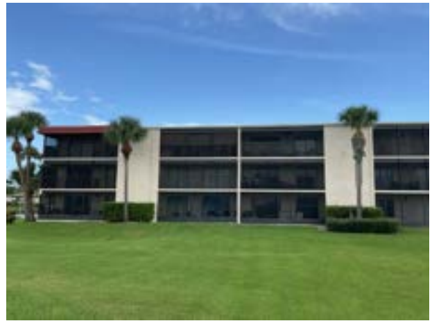
3-story building rear elevation
