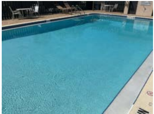
Plaster finish at small pool
