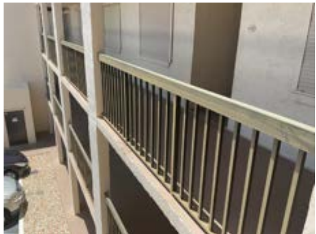
Finish deterioration
