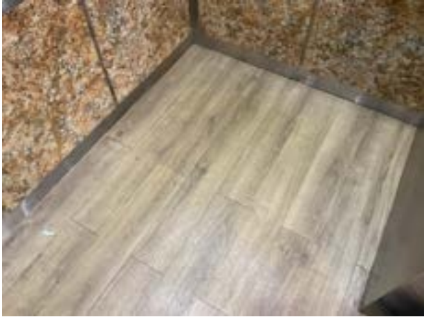
Renovated cab floor finishes
