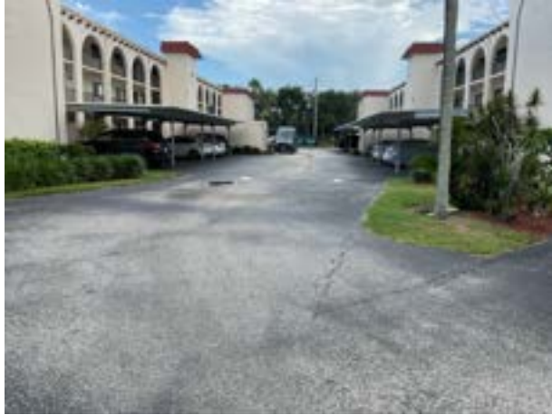
Pavement at 3 story buildings
