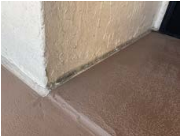
Sealant deterioration
