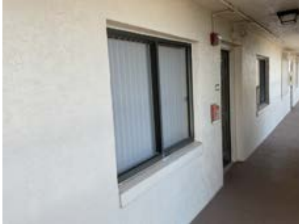
Window at breezeway
