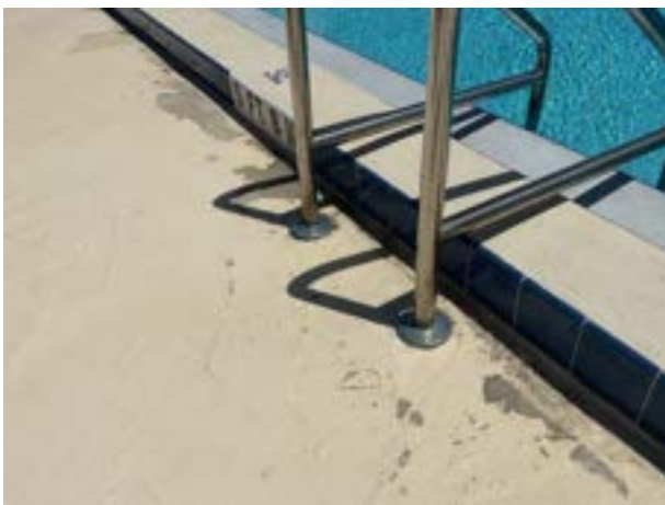
Finish deterioration
