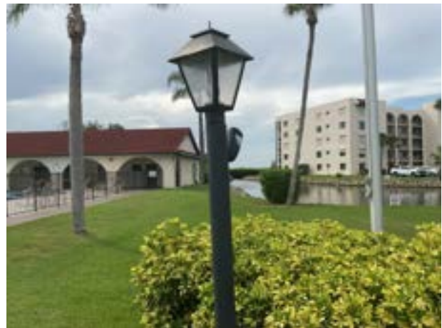
Light pole and fixture
