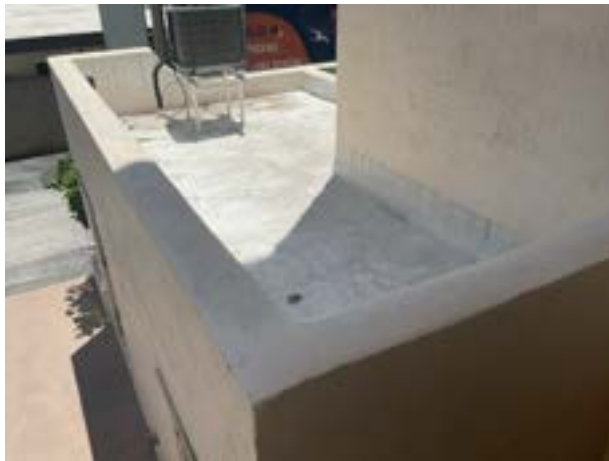
Foam roof overview
