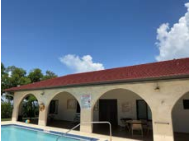
Metal roof at clubhouse
