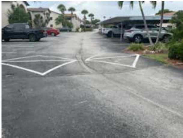
Pavement at 2 story buildings
