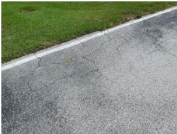
Pavement cracks
