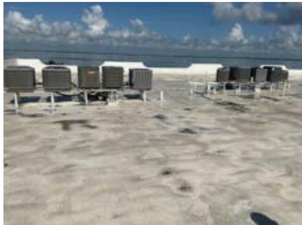
Foam roof overview
