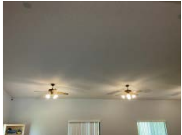
Ceiling and light fixtures
