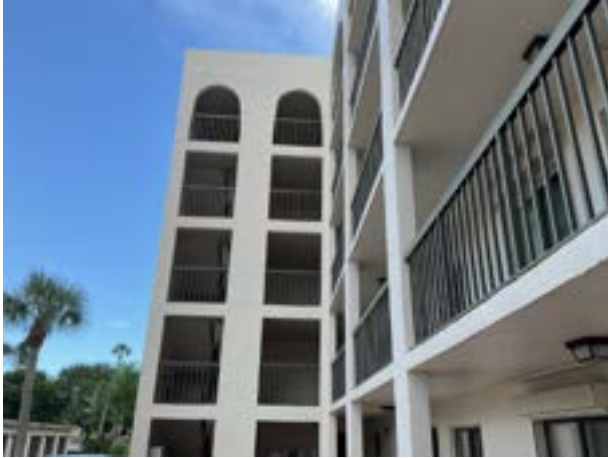
Stucco wall finishes
