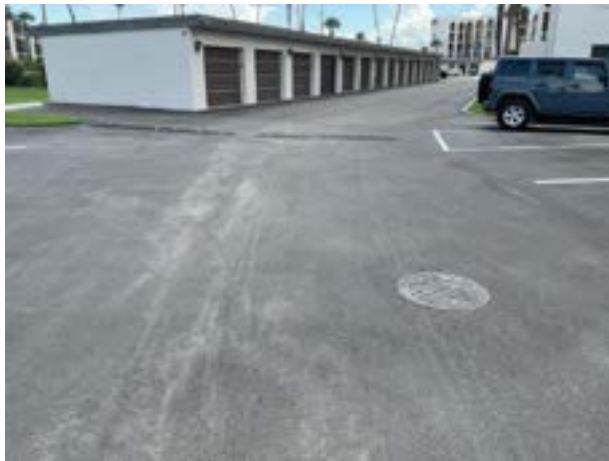
Pavement at 5 story buildings 10-12
