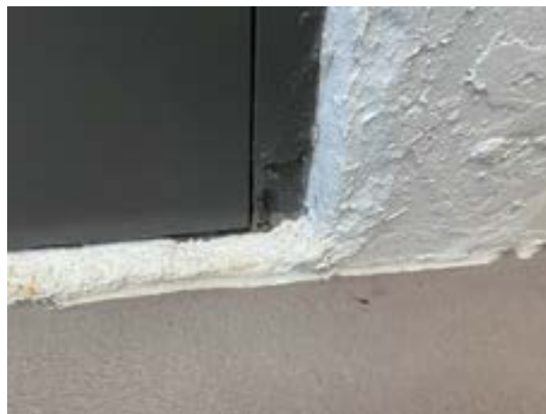
Frame deterioration
