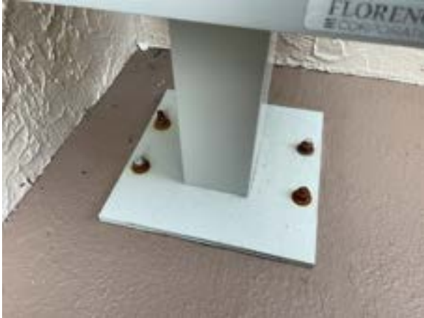
Rusted fasteners
