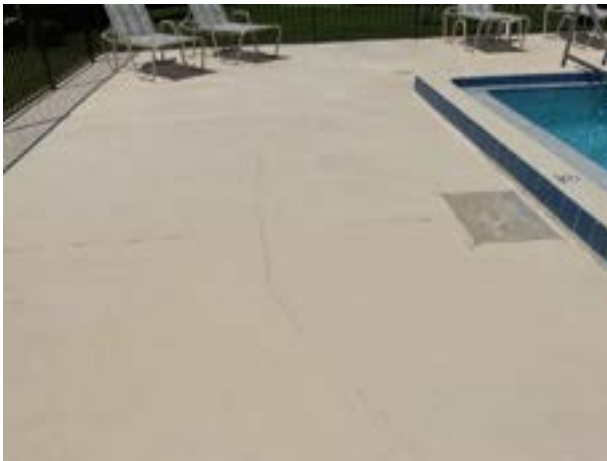
Concrete cracks
