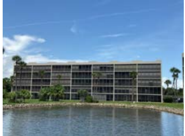
5-story building rear elevation
