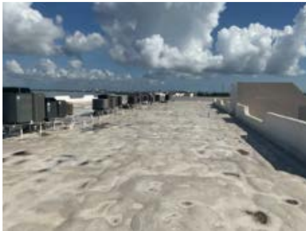
Foam roof overview
