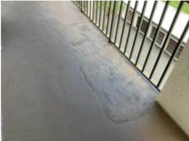
Evidence of partial replacement
