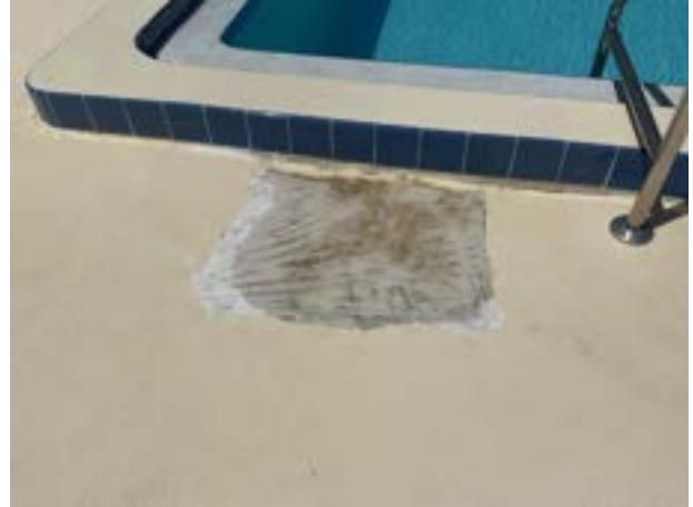
Evidence of ongoing repairs
