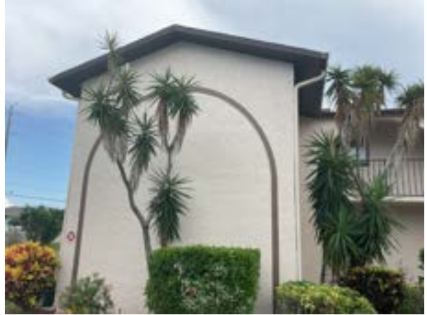
Stucco wall finishes
