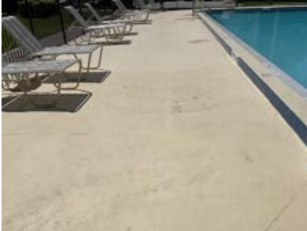
Concrete pool deck overview
