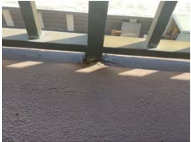
Railing post embedded in concrete
