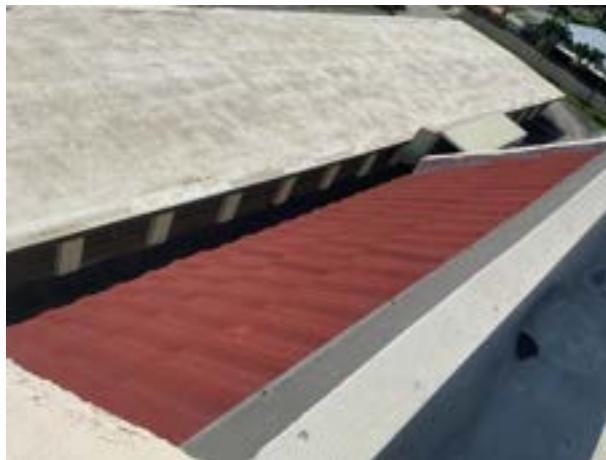
Metal tile roof with coating
