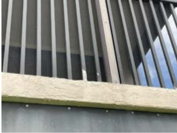
Railing finish fade
