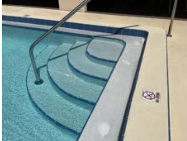
Plaster and tile at steps
