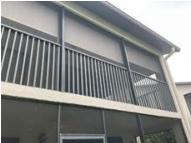
Balcony railings with integrated screen frame
