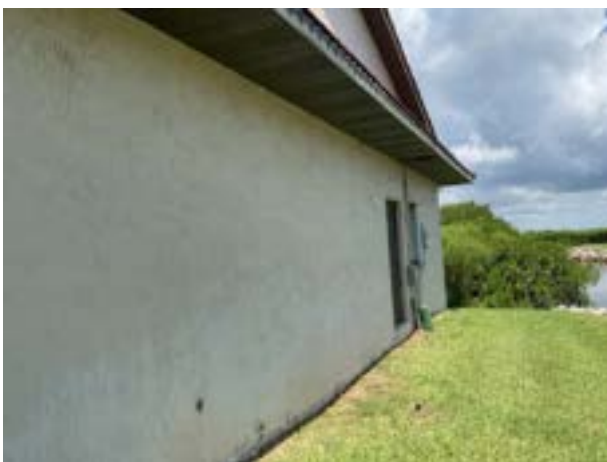
Stucco wall finishes at clubhouse
