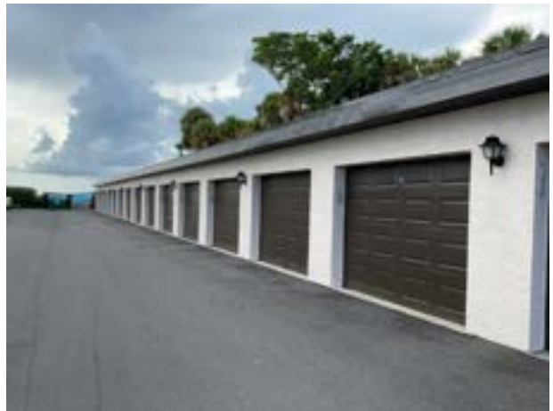
Stucco wall finishes
