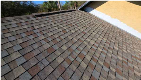
Photos of Each Slope
