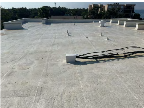
Modified bitumen roof overview
