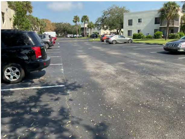
Asphalt pavement overview
