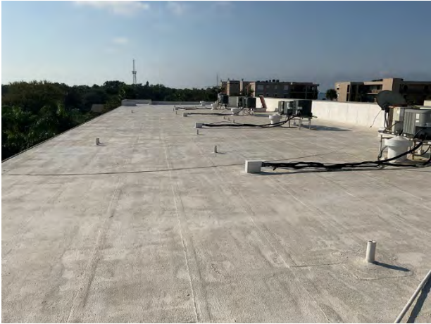
Modified bitumen roof overview
