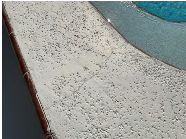
Coping cracks
