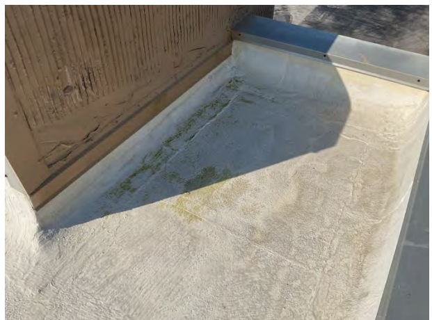
Coating deterioration
