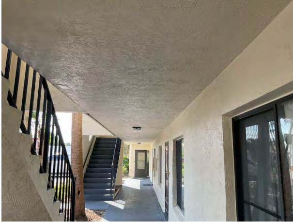
Stucco wall finishes
