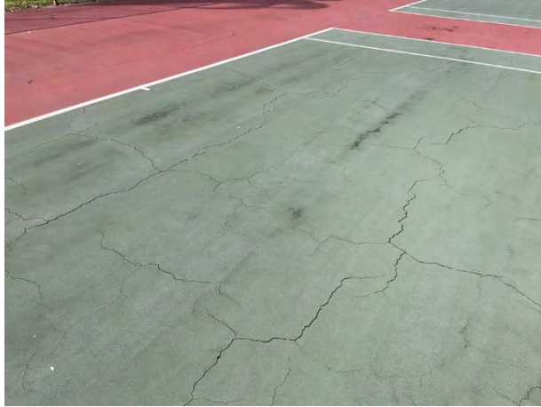
Surface cracks
