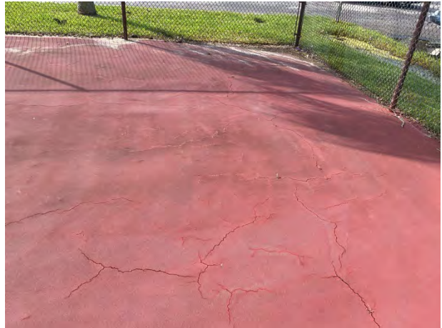
Surface cracks
