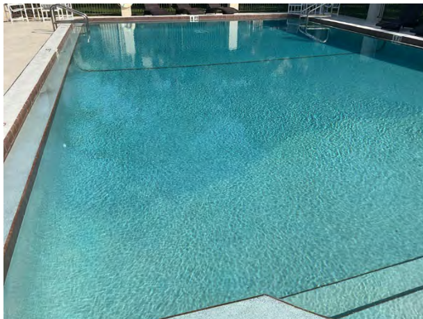
Pool plaster overview
