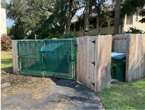
Fences at trash corral overview
