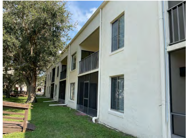
Stucco wall finishes
