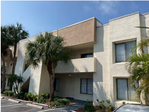
Stucco wall finishes
