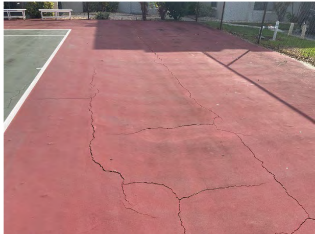
Surface cracks
