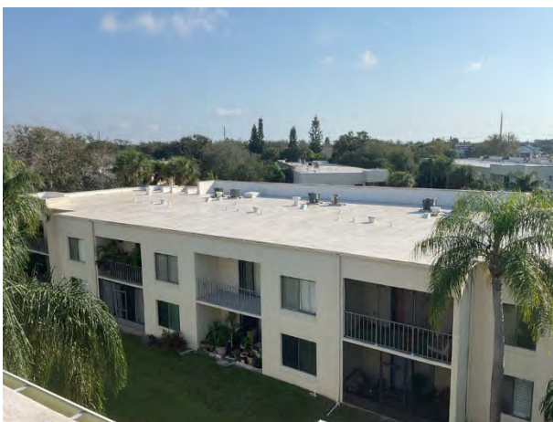
Modified bitumen roof overview
