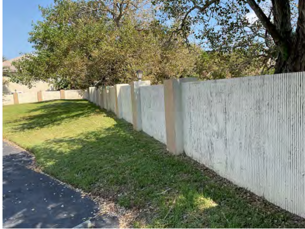
Perimeter wall overview
