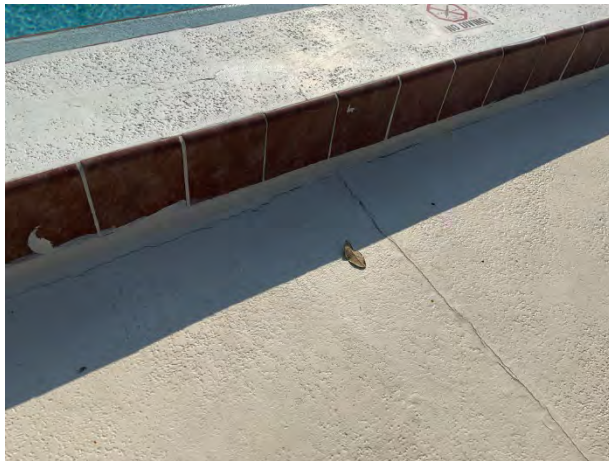
Concrete cracks
