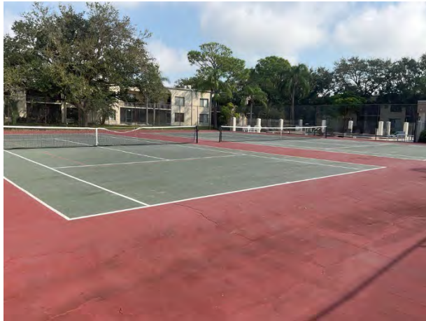
Tennis court overview
