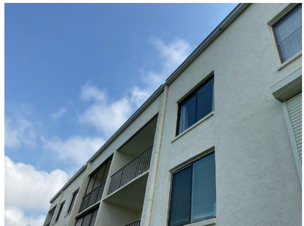
Metal gutters and downspouts
