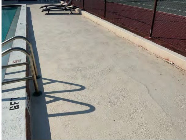
Concrete deck overview
