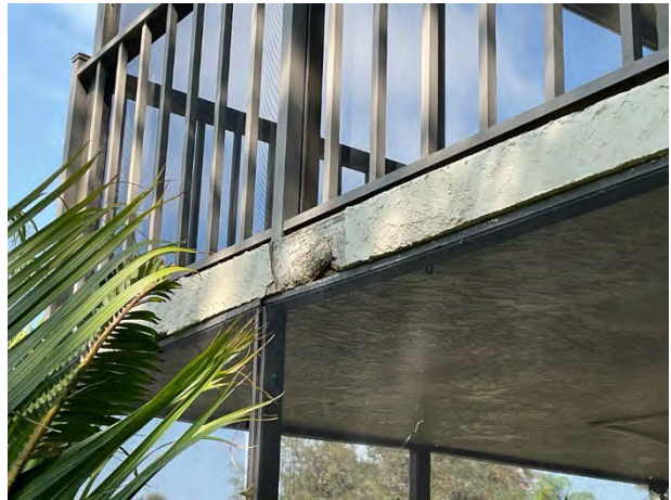
Exposed reinforcement
