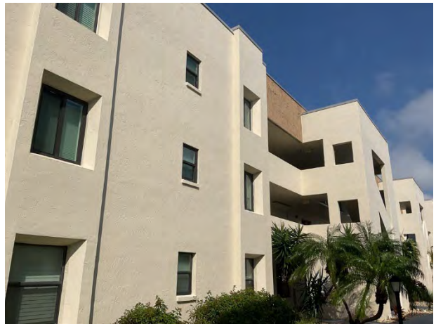
Stucco wall finishes
