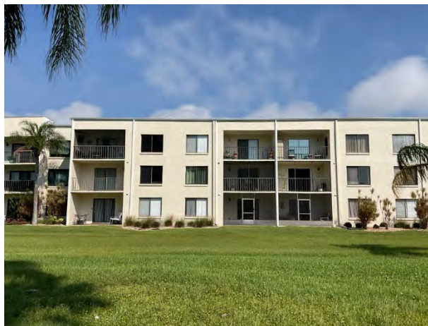
Typical three story building rear elevation
