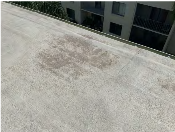
Coating deterioration
