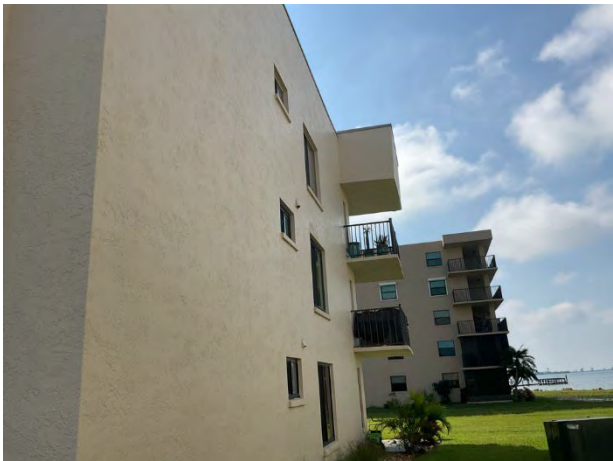
Stucco wall finishes
