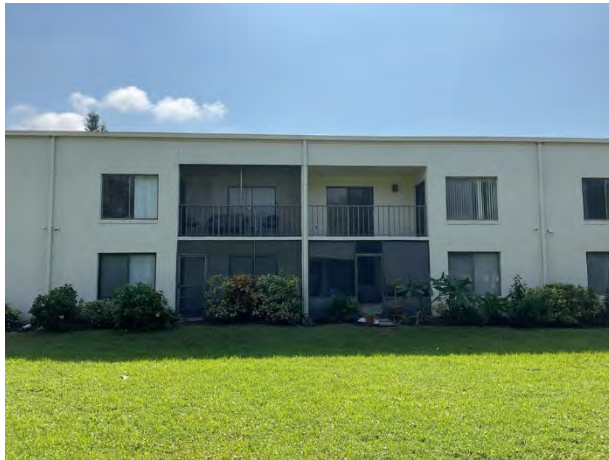
Typical two-story building rear elevation
