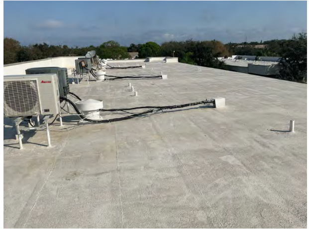
Modified bitumen roof overview
