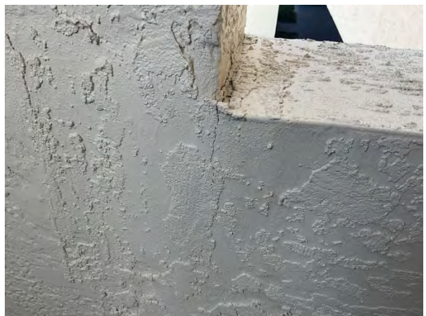
Stucco cracks
