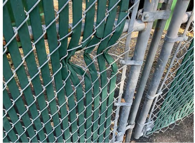
Fence warped webbing
