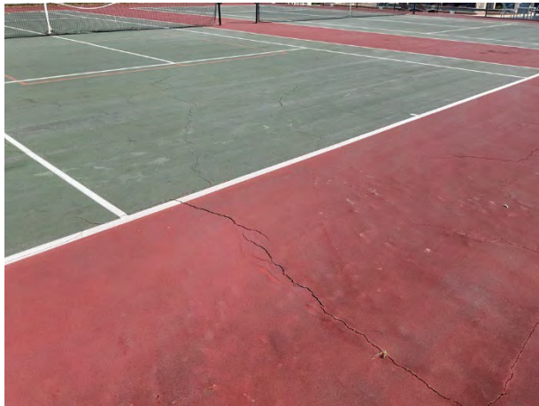
Surface cracks
