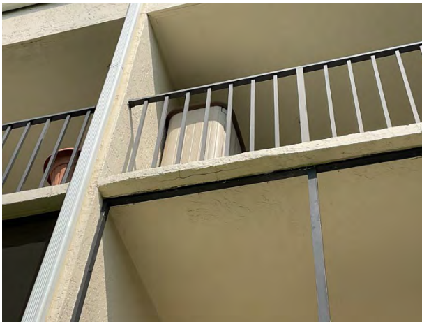
Concrete cracks
