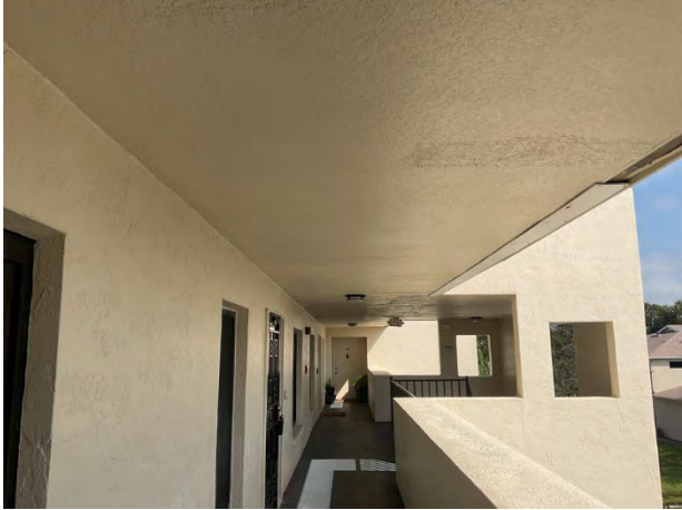
Stucco wall finishes
