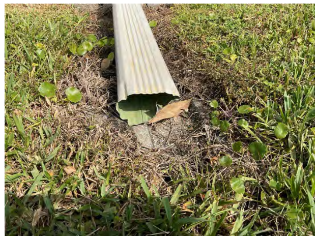
Downspout damage
