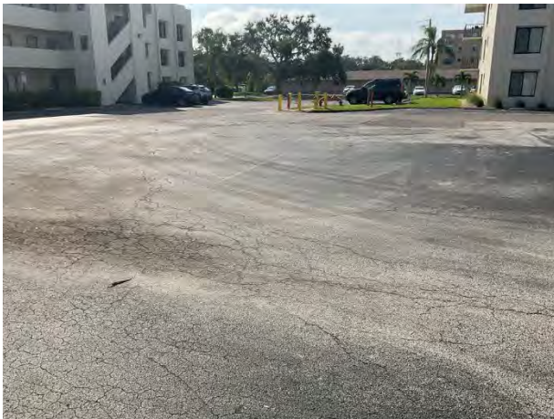
Asphalt pavement overview
