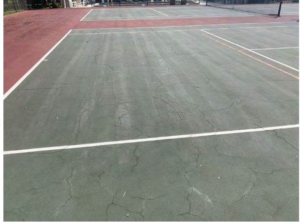
Surface cracks
