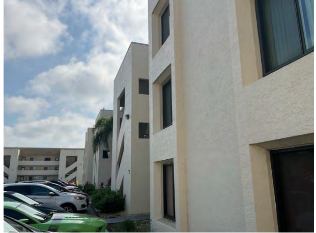
Stucco wall finishes
