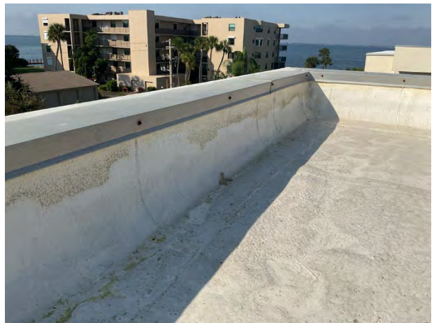
Coating deterioration
