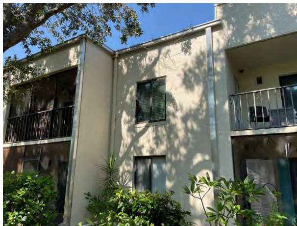
Aluminum gutters and downspouts
