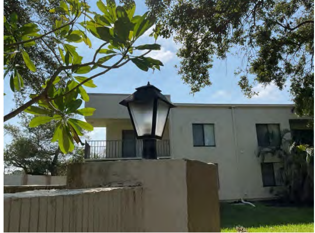
Wall light fixture
