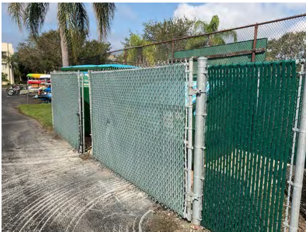
Fences at trash corral overview
