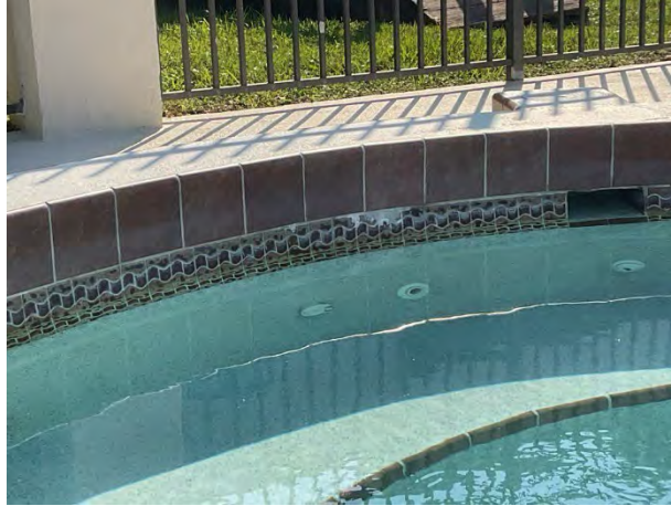
Tile deterioration
