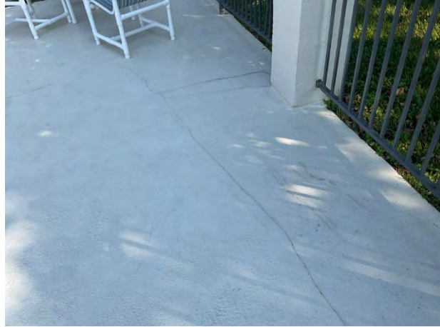
Concrete cracks
