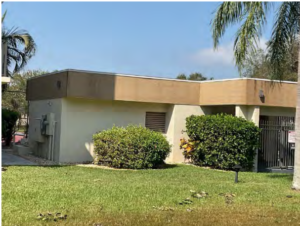
Stucco wall finishes at pool house
