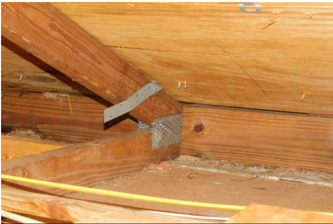
TRUSS TO WALL CONNECTION
