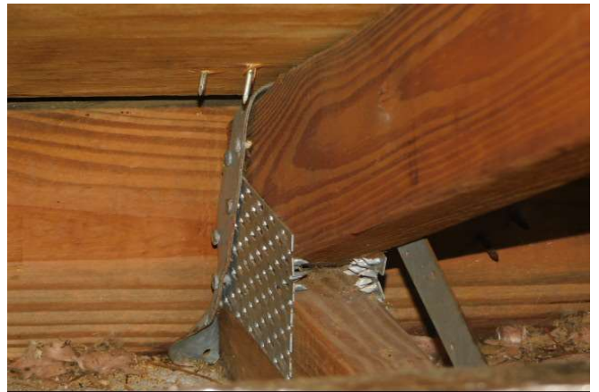
TRUSS TO WALL CONNECTION
