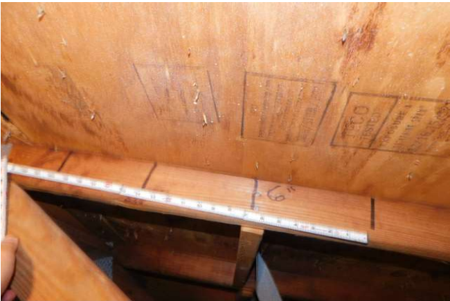
ROOF DECK ATTACHMENT SPACING
