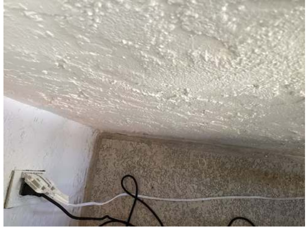
Sealant at balcony perimeter
