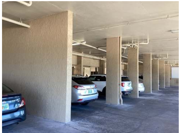
Concrete columns at center tower garage
