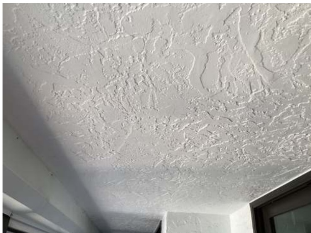
Unit 304 balcony underside
