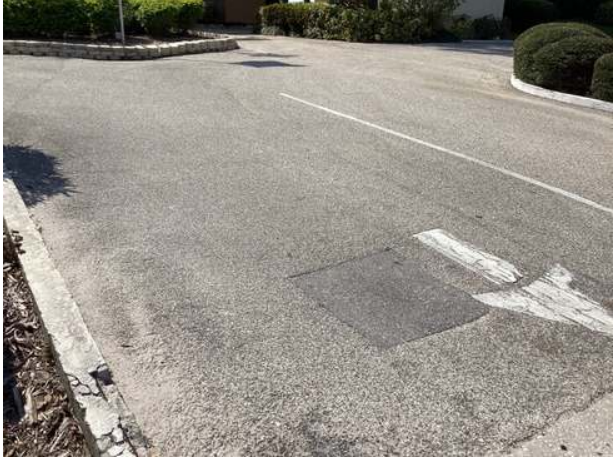
Asphalt pavement entrance overview with patch
