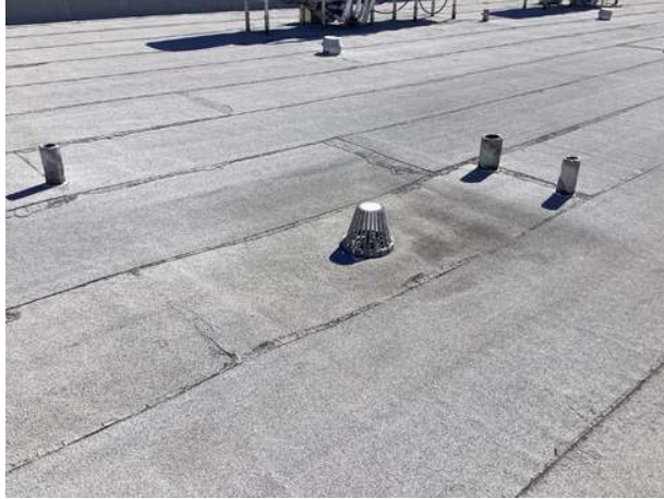
South tower roof drain
