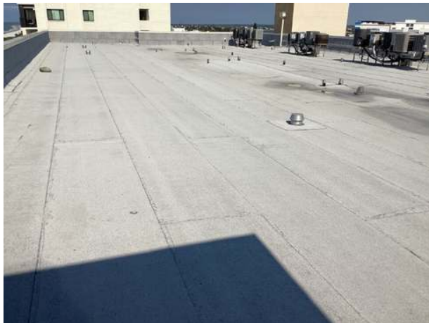
Modified bitumen roof overview
