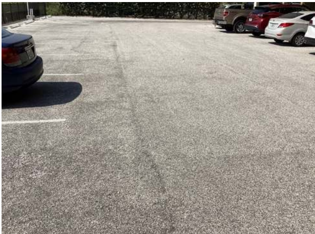
Asphalt pavement parking lot overview
