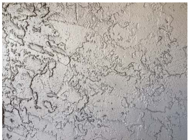
Stucco wall finishes
