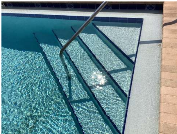
Pool plaster finish with tile perimeter
