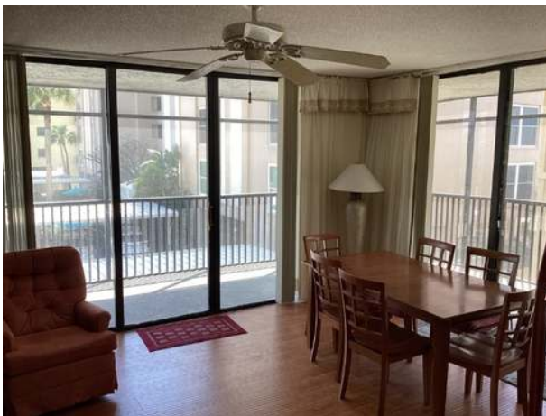
Sliding glass doors at the common unit
