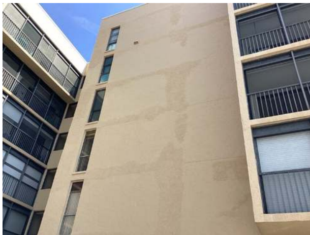
Previous stucco repairs
