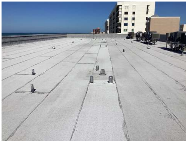
Center tower modified bitumen roof overview
