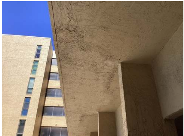
Undersides of south tower first floor balconies
