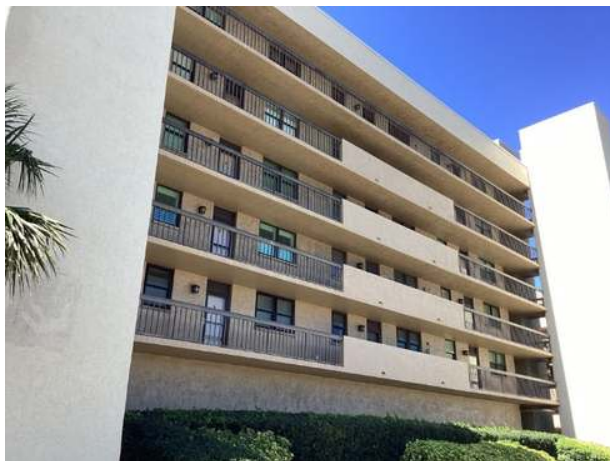
South tower east elevation
