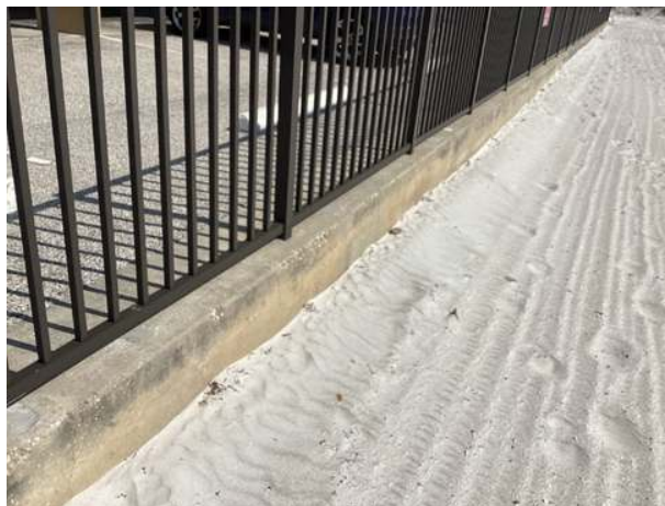
Concrete bulkhead overview
