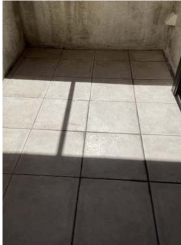
Unit 201 Balcony overview
