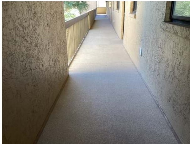
Third floor breezeway at center tower
