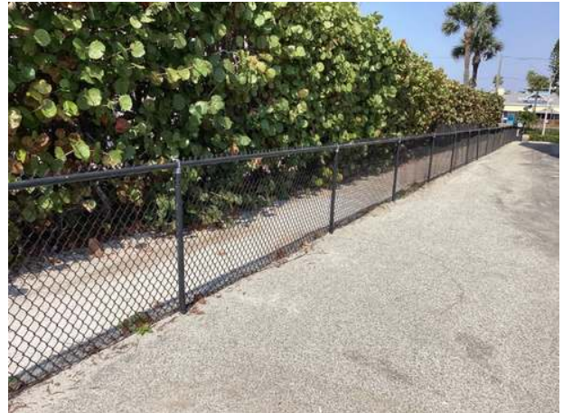
Chain link fence at northwest perimeter
