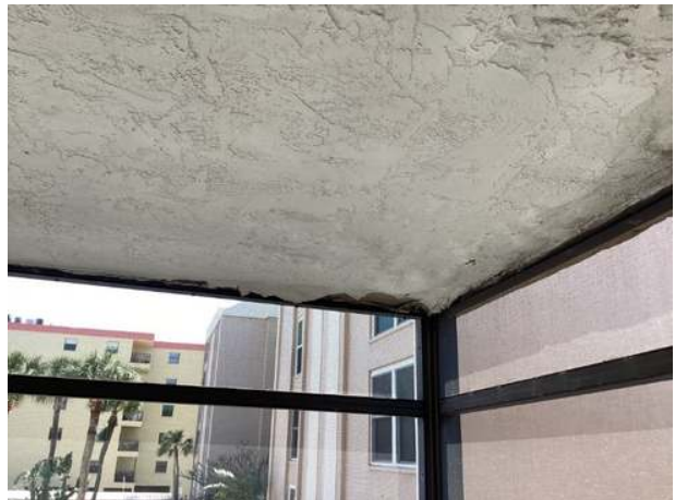
Common unit balcony ceiling
