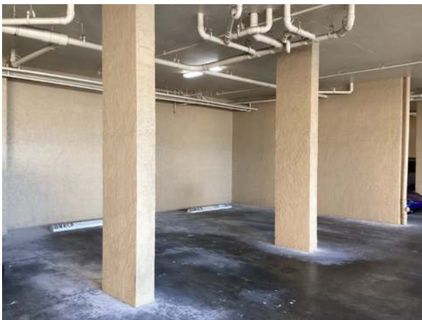
Stucco wall finishes at garage
