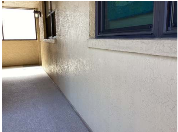
Stucco wall finishes at third floor center tower
