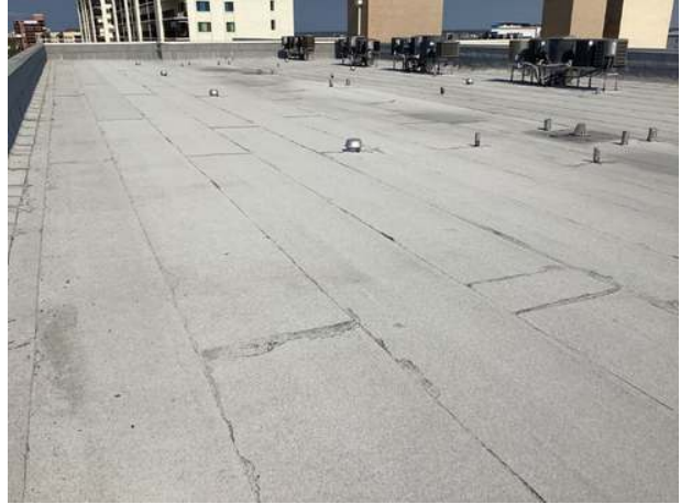
Modified bitumen roof overview
