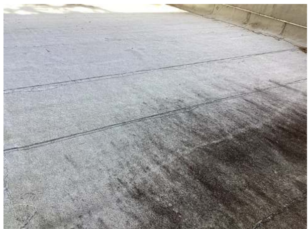
Modified bitumen roof at the lobby
