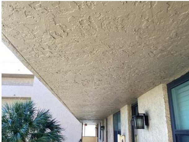
Fourth floor breezeway underside at center tower
