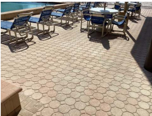
Paver pool deck overview
