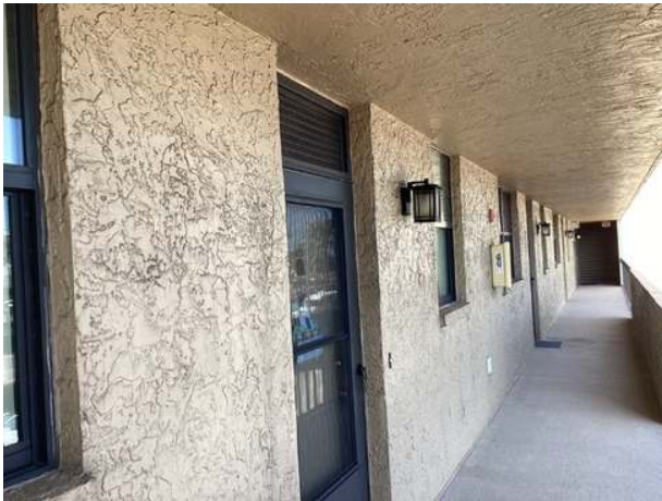
Stucco wall finishes at breezeway
