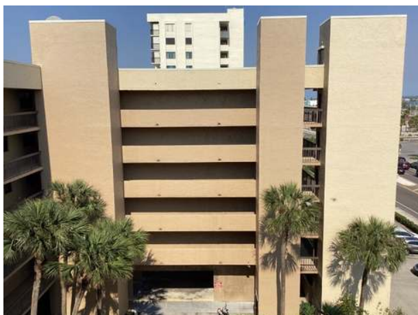
Stucco wall finishes
