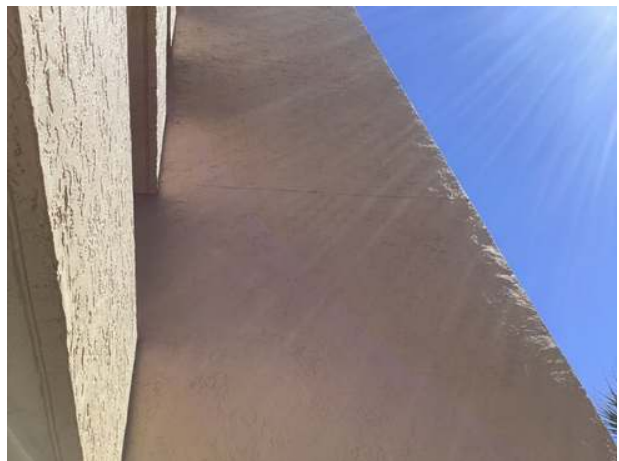
Stucco wall finishes at north tower trash chute
