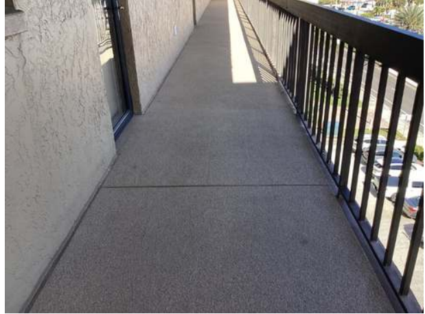
5th floor north tower breezeway
