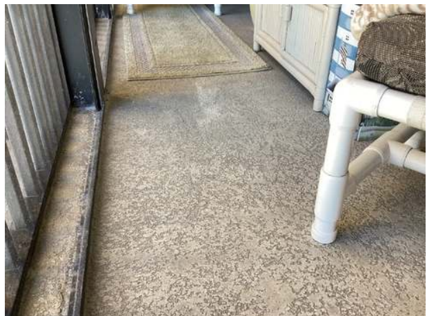
Concrete balcony at unit 204
