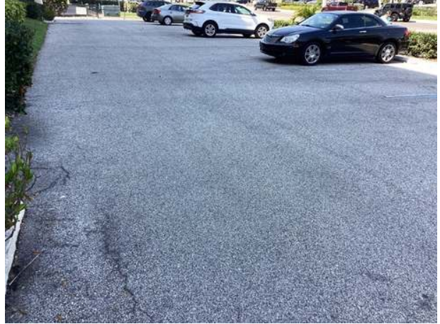
Asphalt pavement parking lot overview
