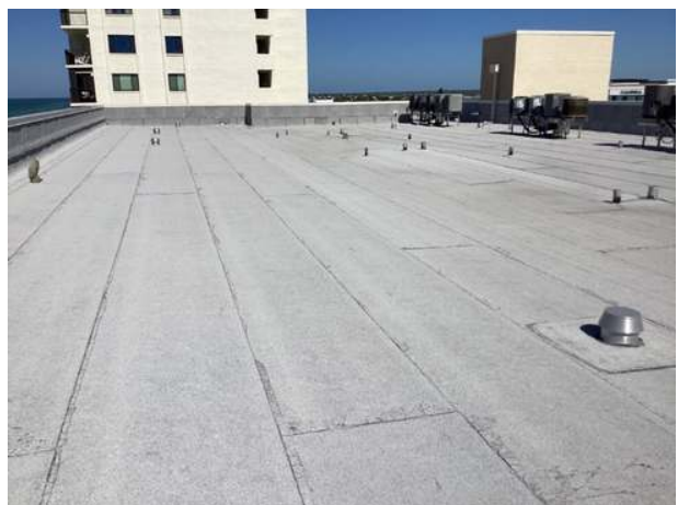
South tower modified bitumen roof overview
