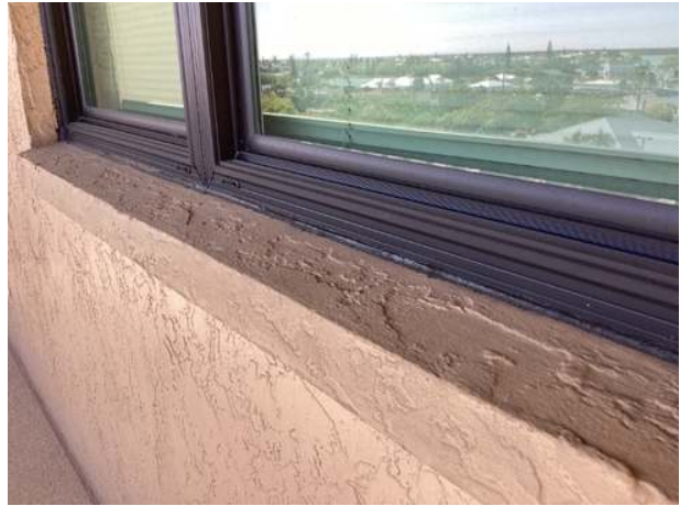
Sealant in good condition at unit 412 front window Sealant in good condition at unit 509 front window
