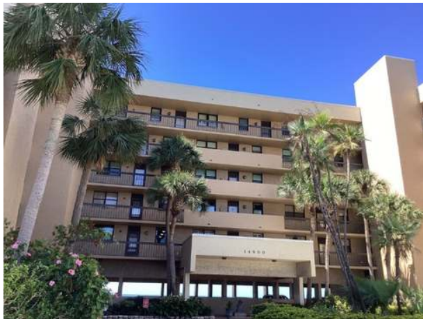
Center tower east elevation
