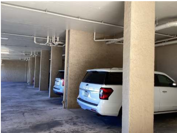
Columns at north tower garage
