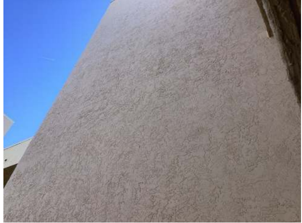
Stucco wall finishes at south tower elevator
