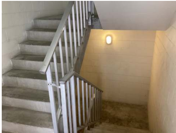
Stairwell paint finishes
