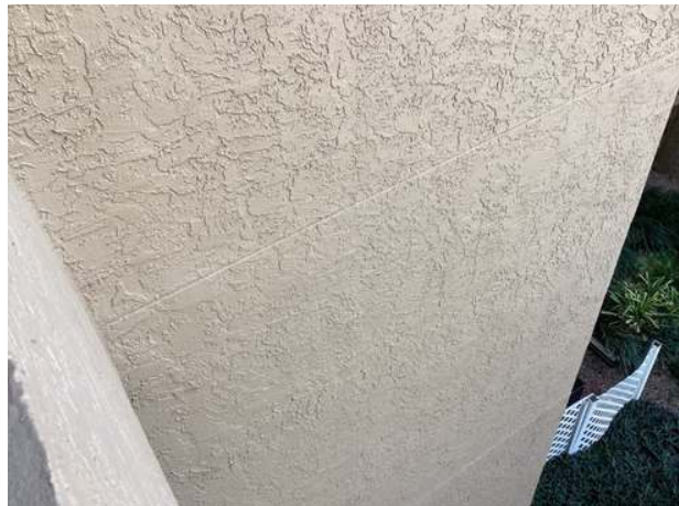
Stucco wall finishes
