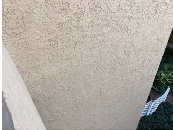
Stucco wall finishes
