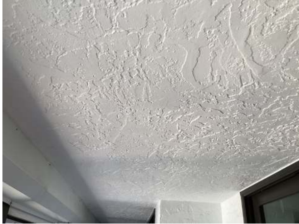
Unit 304 balcony underside
