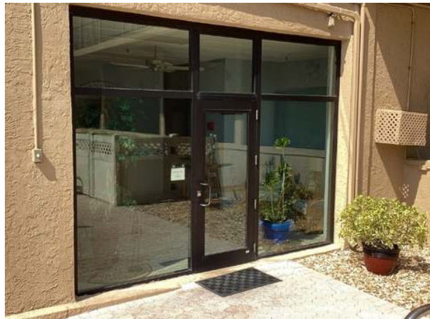
Common windows and door at lobby
