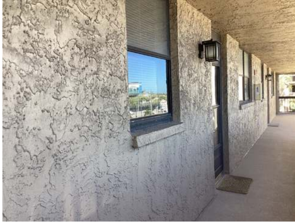
Stucco wall finishes at second floor south tower
