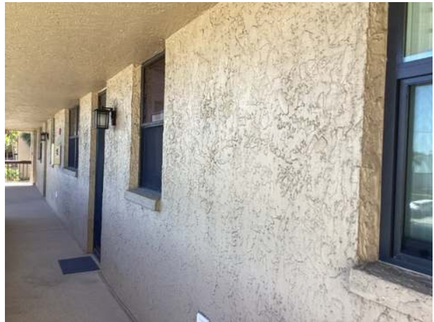
Stucco wall finishes at first floor north tower
