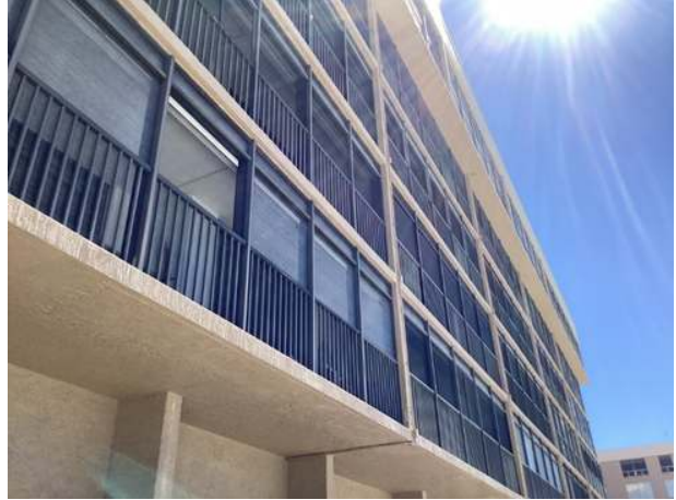
Center tower balconies
