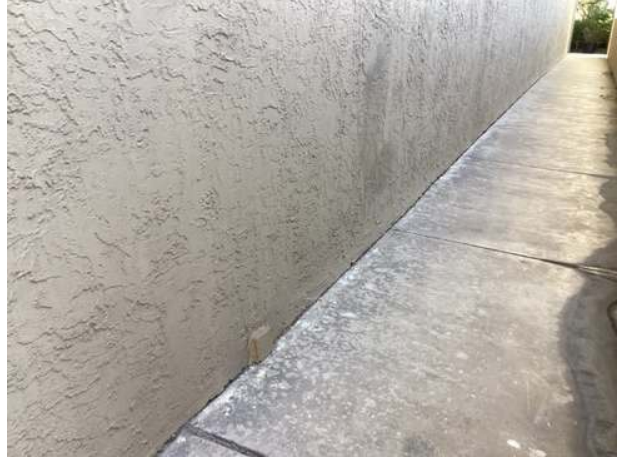
Stucco terminates at grade
