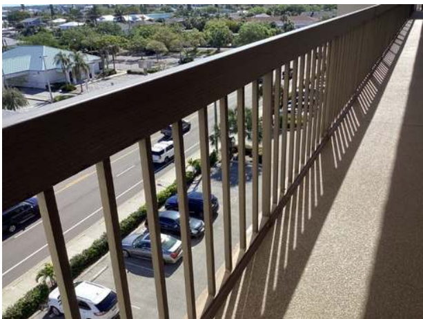
Aluminum railings at north tower 5th floor breezeway
