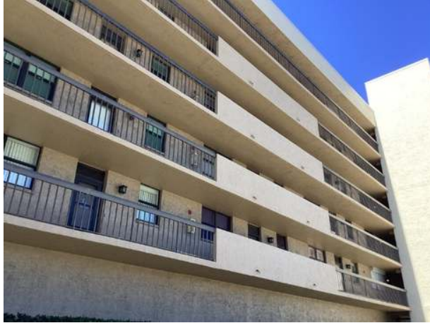
North tower breezeway overview
