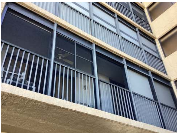
Aluminum railings and screens at north tower first floor balconies
