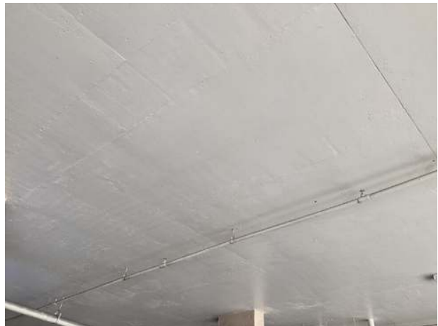
Underside of center tower first floor
