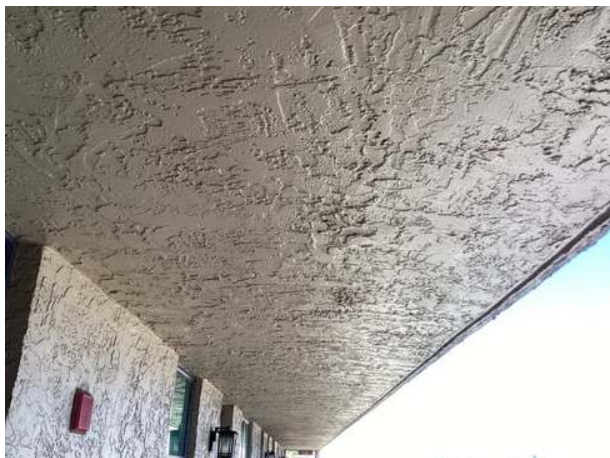
Underside of third floor south tower breezeway
