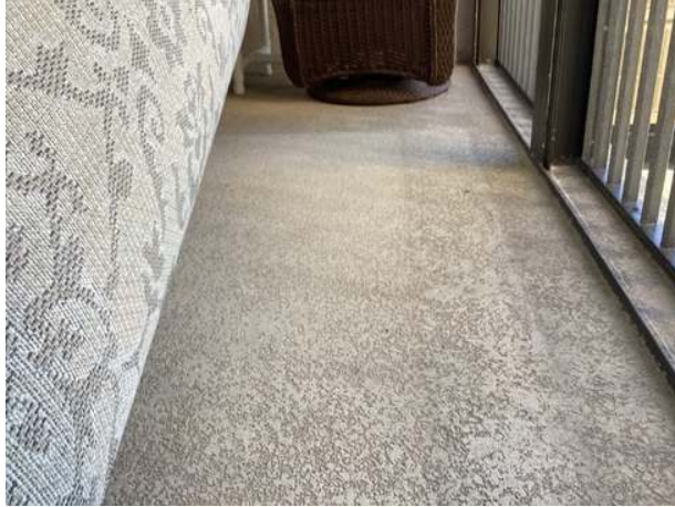
Concrete balcony at unit 204
