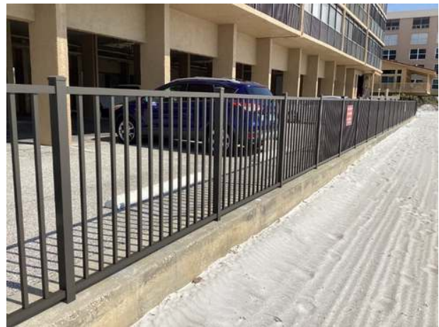
Aluminum fence at southwest perimeter
