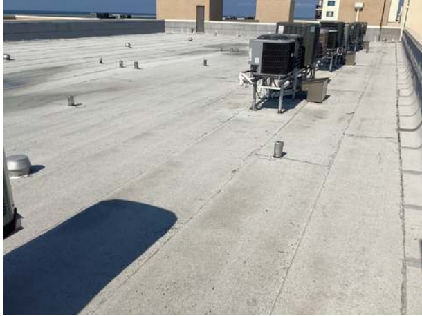
Modified bitumen roof overview
