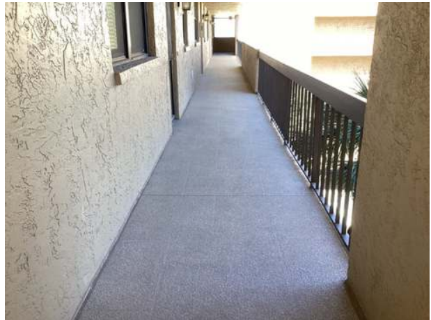
Fourth floor center tower breezeway
