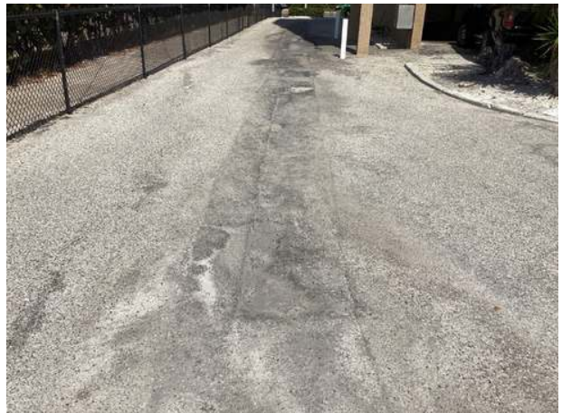
Pavement deterioration
