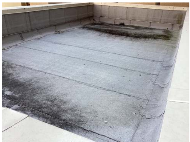
Modified bitumen roof overview at first floor
