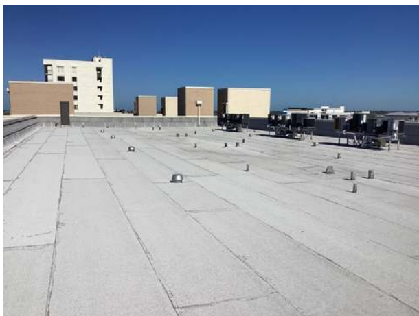
South tower modified bitumen roof overview
