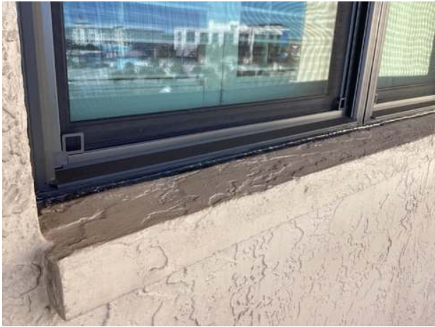
Sealant in good condition at unit 412 front window Sealant in good condition at unit 509 front window
