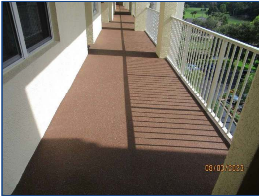
Photograph No. 39: General view of the exterior walkway.
