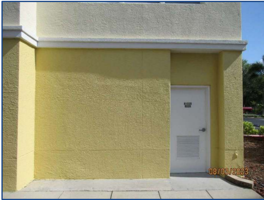
Photograph No. 41: General view of a common door.
