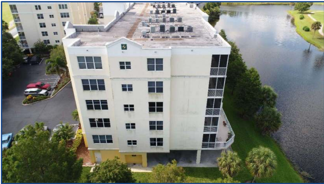
Photograph No. 2: North elevation.
