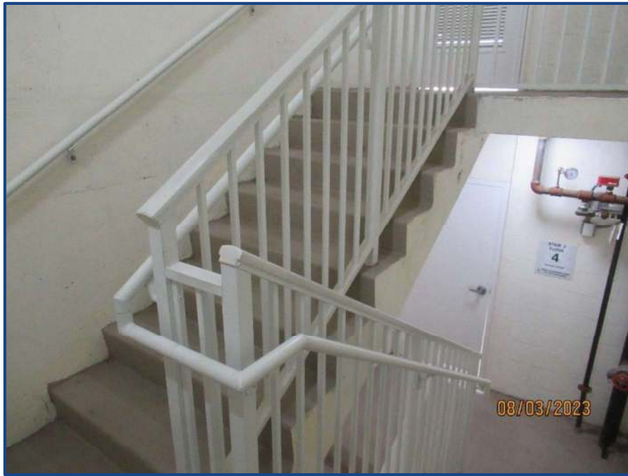
Photograph No. 21: General view of the cast in place concrete stairs.
