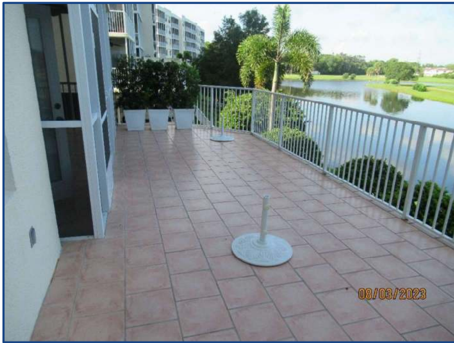
Photograph No. 12: Exterior balcony of Unit 6101.
