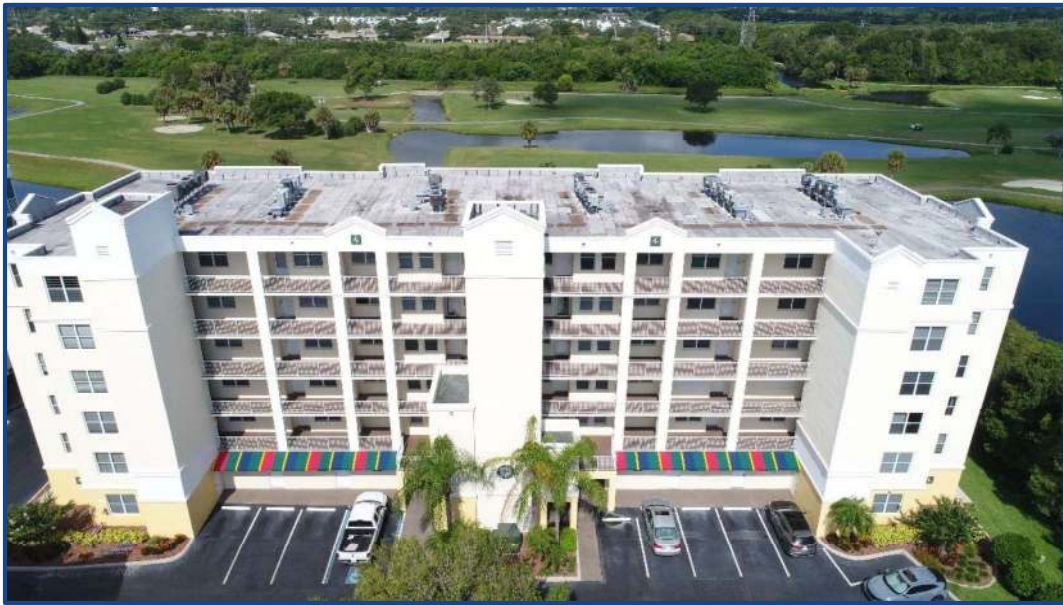
Photograph No. 1: East (front) elevation.
