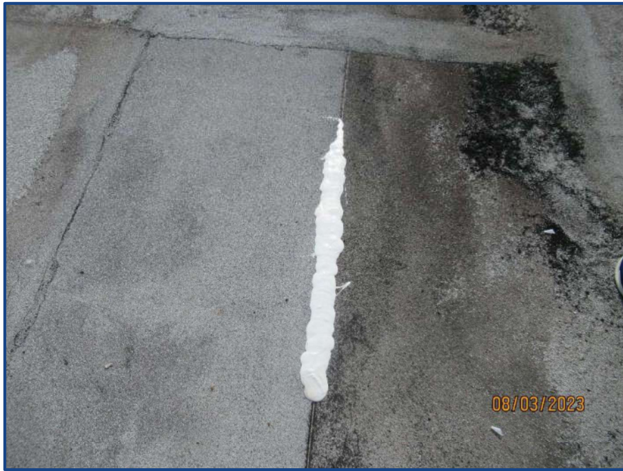
Photograph No. 19: View of previous roof patch repair.
