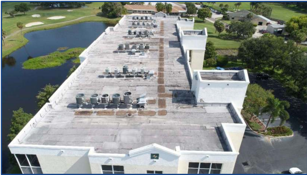
Photograph No. 5: Roof.
